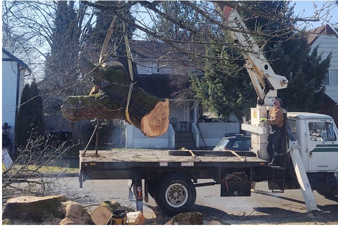
Hazardous tree removal in McKinley
